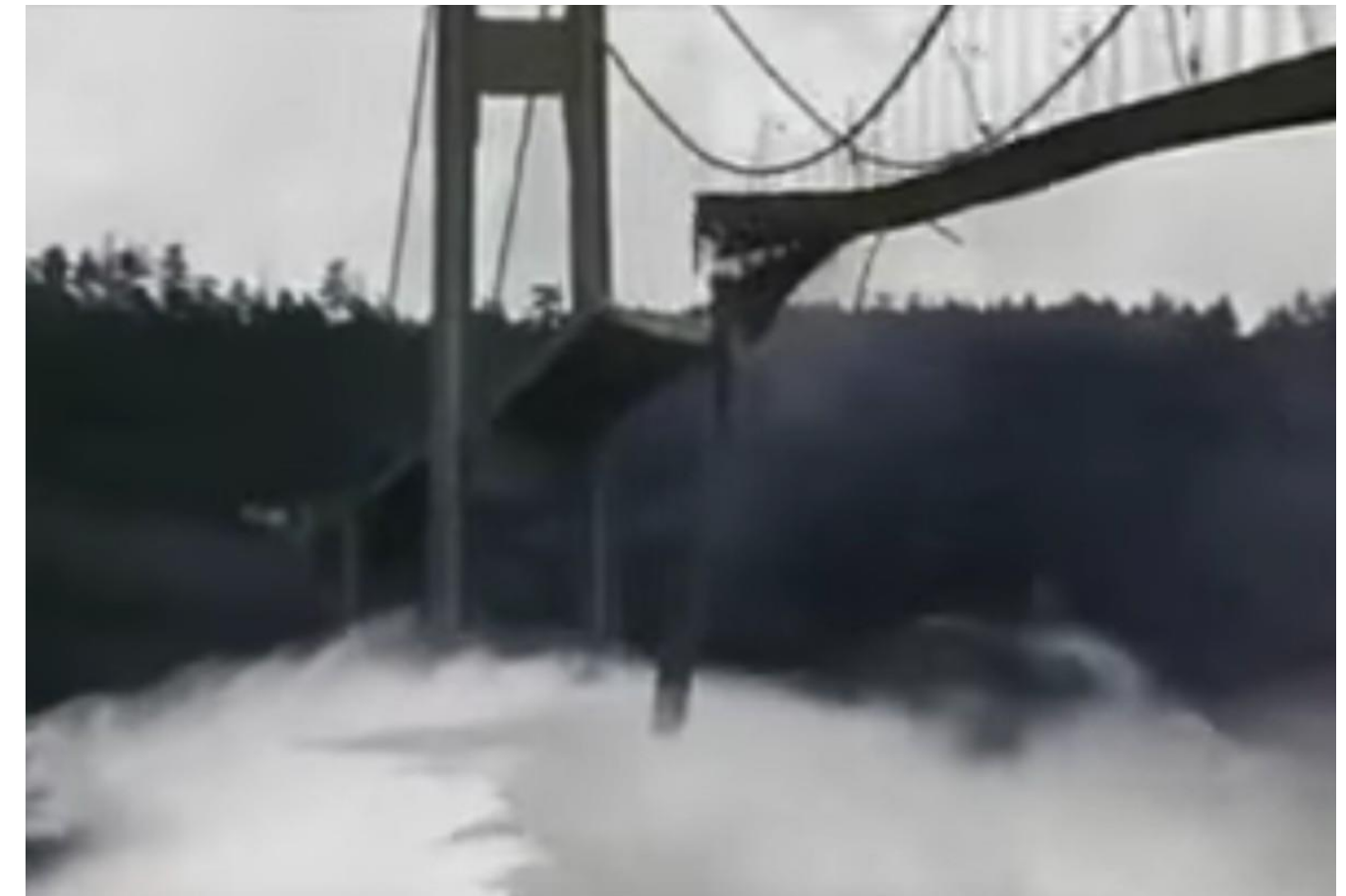
Tacoma Narrows Bridge
