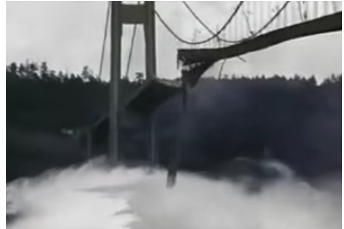
Tacoma Narrows Bridge
